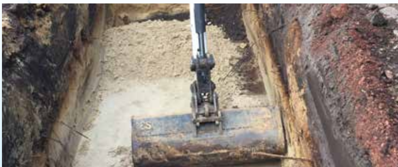
Gat graven, bodem wit zand
